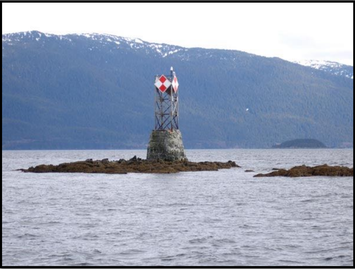
Figure 5: A modern navigation aid now sits atop Vanderbilt Reef in the Lynn Canal fjord just north of Juneau, Alaska. Look for the beacon on your next Alaskan cruise up the inside passage.
